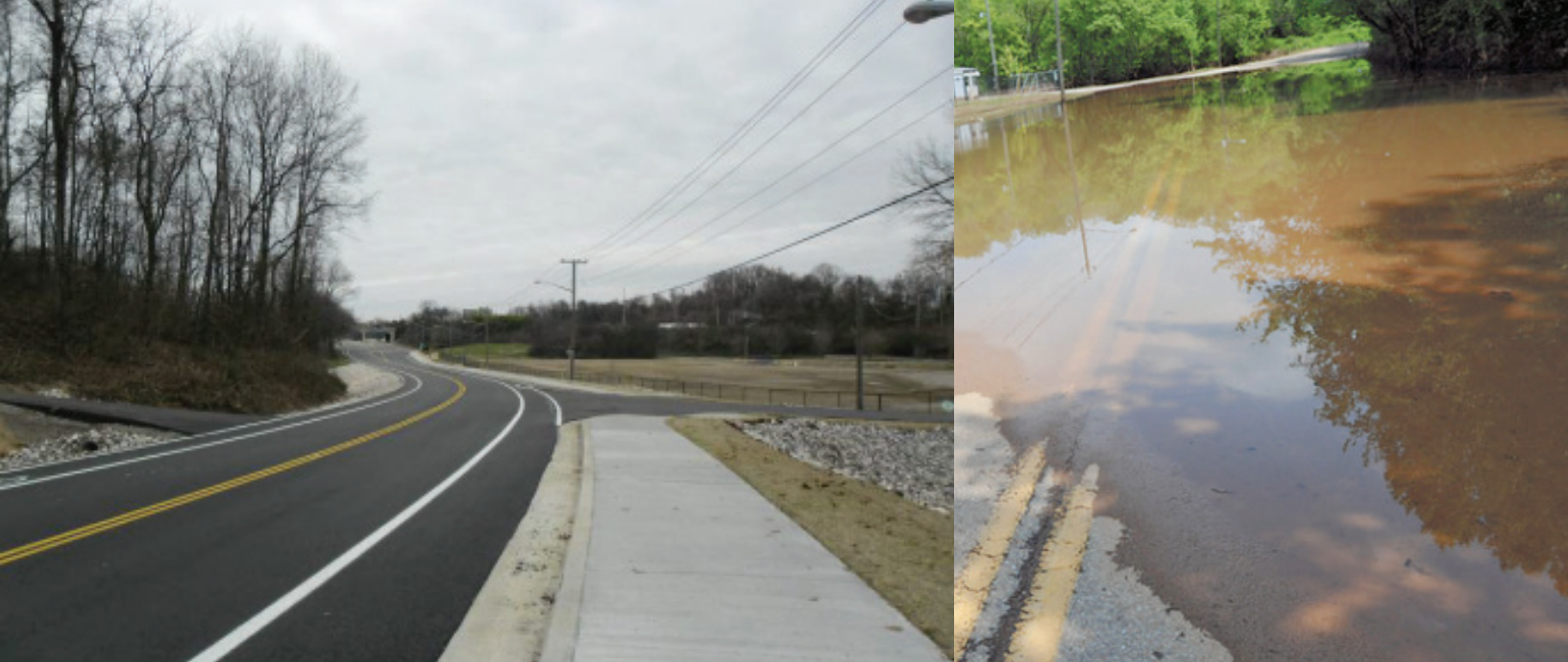
Photos above: The reconstruction of about 1,600 feet of Prosser Rd between Knoxville Zoo Drive and East Magnolia Ave was necessary to reduce flooding, which for many years had regularly shut down the road. The reconstruction not only raised the road, but also added bicycle lanes. Photos courtesy of (left) City of Knoxville and (right) Knoxville News Sentinel.
