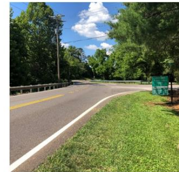
Looking north on Northshore Drive west of Tooles Bend Road
