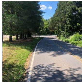
Looking west on Tooles Bend Road towards Northshore Drive
