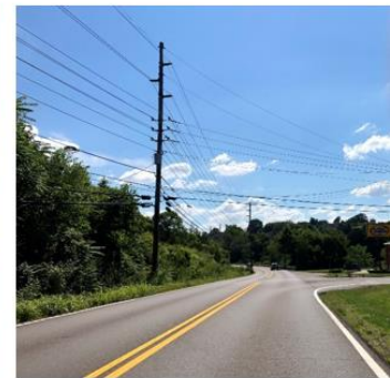
Looking west on Northshore Drive east of Hart Road
