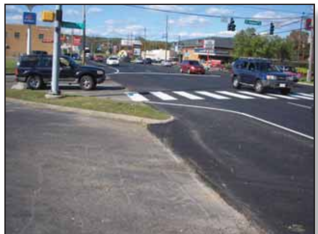
There is no designated bike lane and motorists use the shoulder as a deceleration and turning lane.
