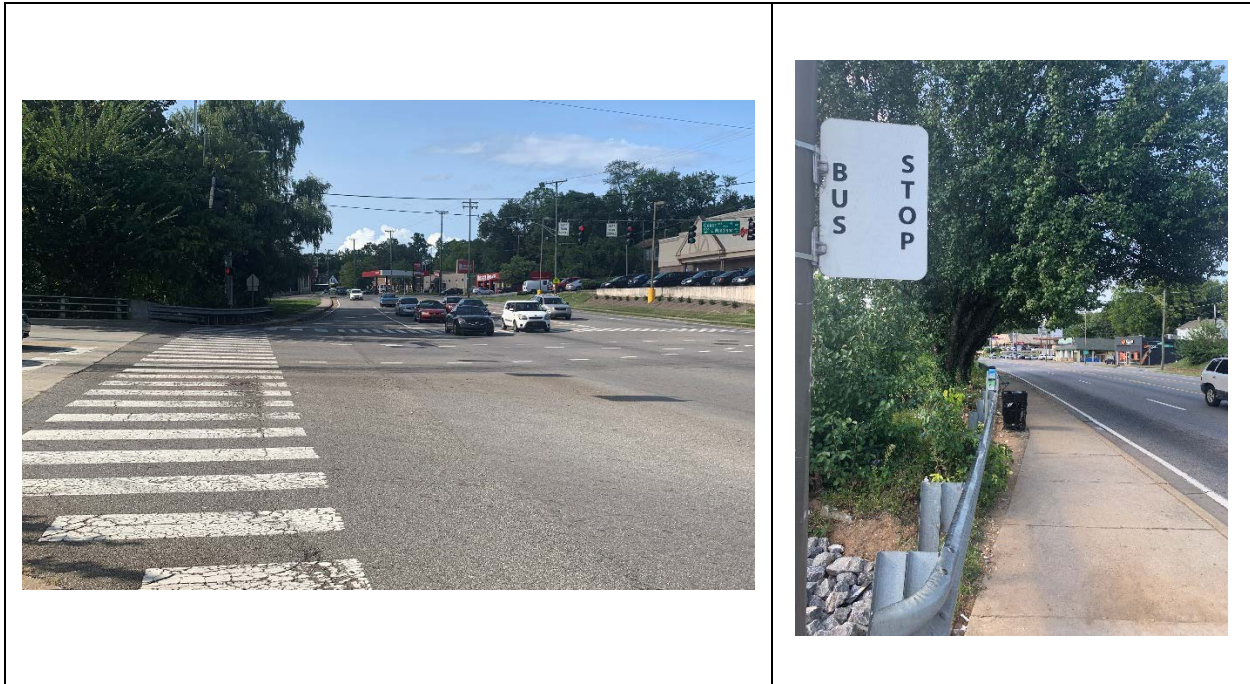
Left Image: A photo of the Woodland Ave/Coker intersection, looking north, showing the wide crossing distances across Broadway. The crossing distance is approximately 100' curb to curb.
