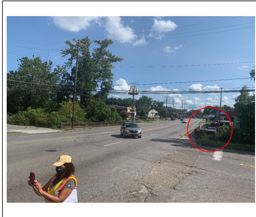
Above Image: A photo, looking south from Chickamauga Ave, showing an uncontrolled intersection and vegetation along the bridge that is reducing pedestrian visibility (red circle). This location was recommended for evaluation for installing a traffic signal.
